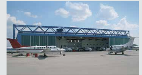
2014 Acquisition of Augsburg Air Service
